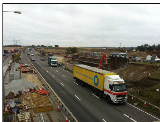
Improvement works at M1 Junction 12
