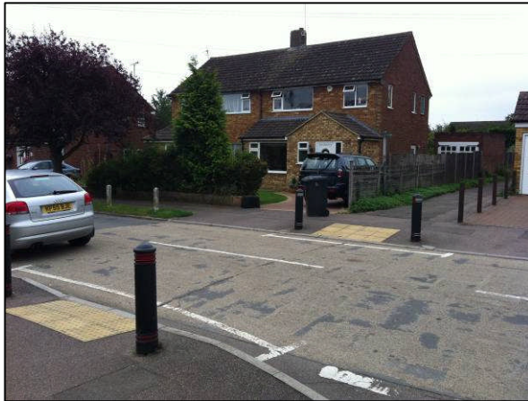
Crossing point with dropped kerb and markings
