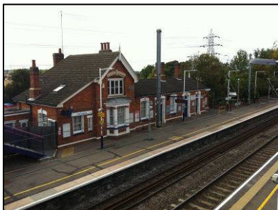
Harlington Rail Station
