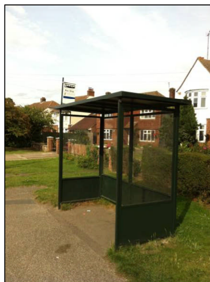
Poor quality bus stop in Barton-le-Clay
