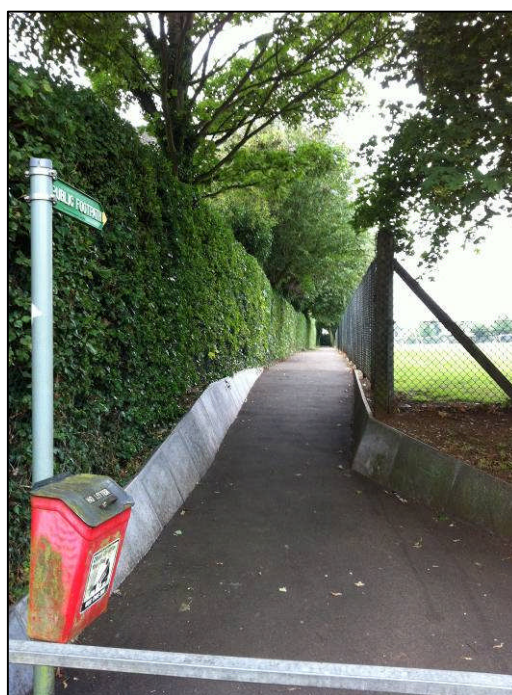
Recently improved footpath in Toddington
